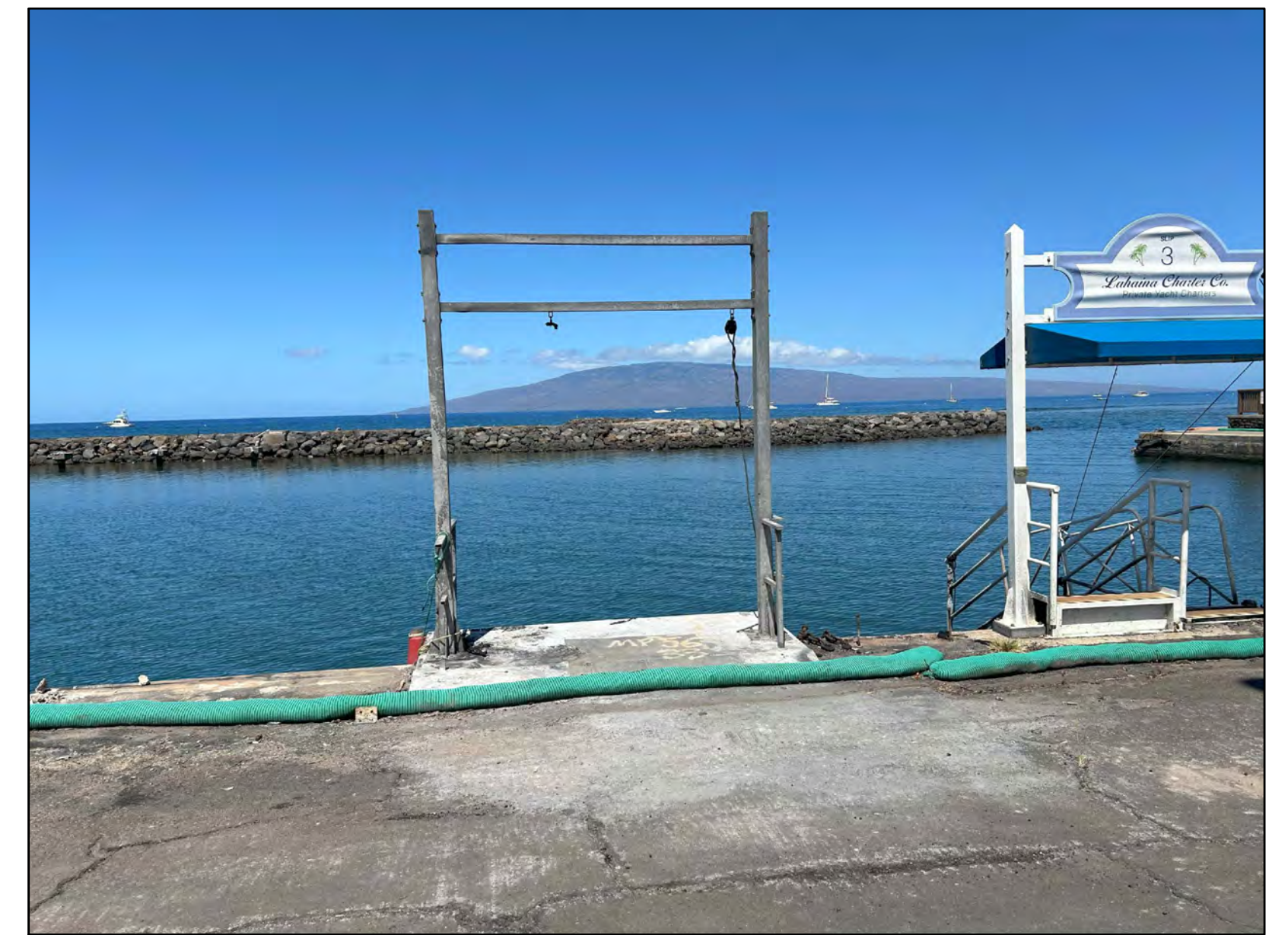
3 EXIST. METAL STRUCTURE TO BE REMOVED TAKEN 06/25/2024
