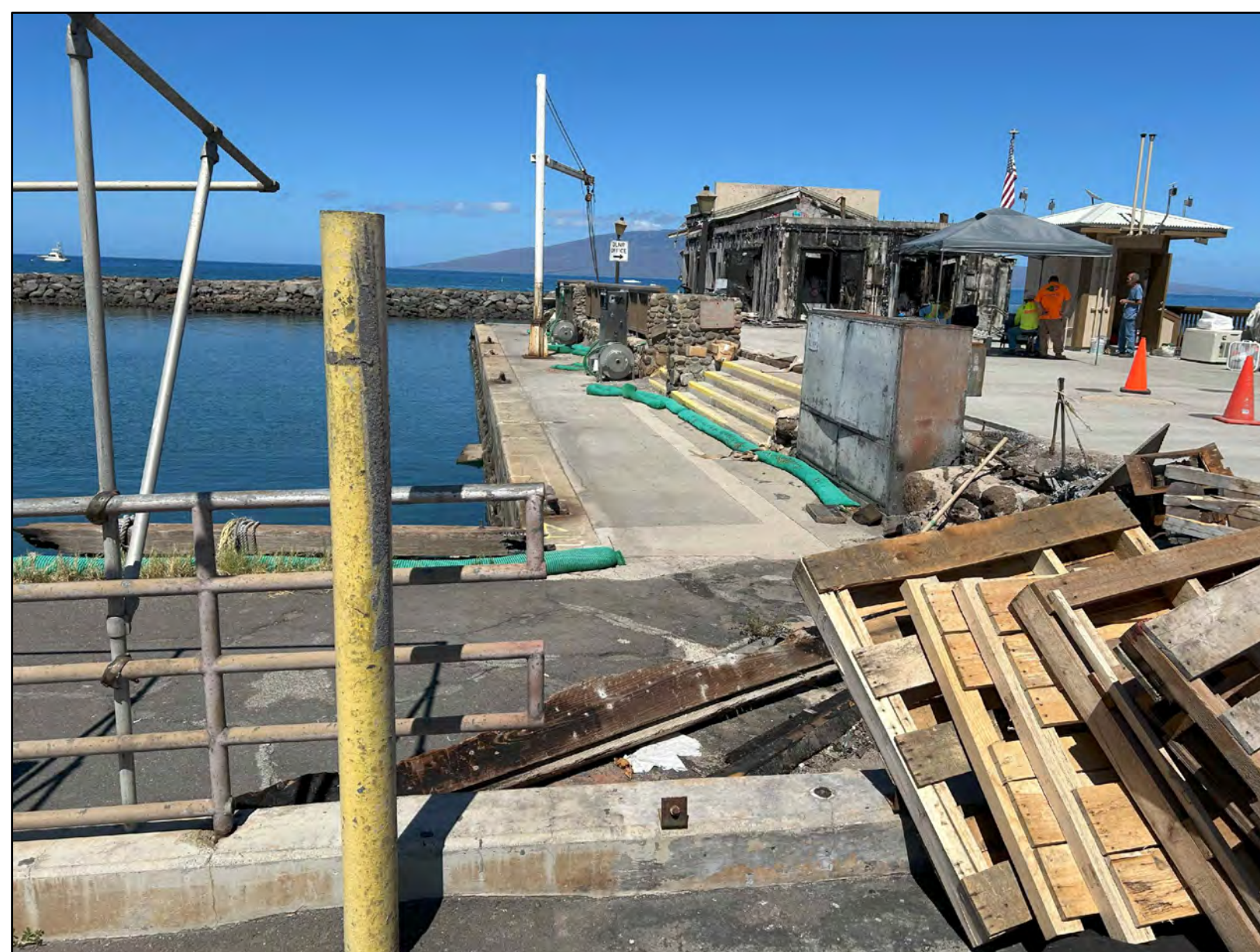
8 EXIST. CONDITIONS OF LAHAINA LOADING DOCK TAKEN 06/25/2024
