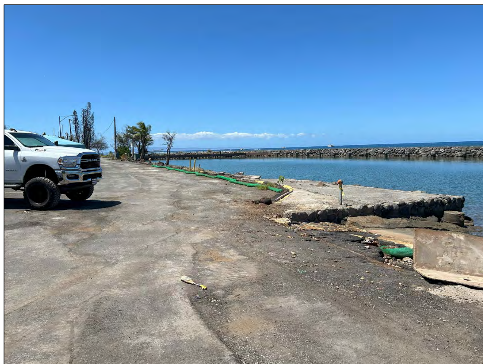
7 EXIST. CONDITIONS ON SOUTHERN SIDE OF LAHAINA SBH, FRONT ROW TAKEN 06/25/2024
