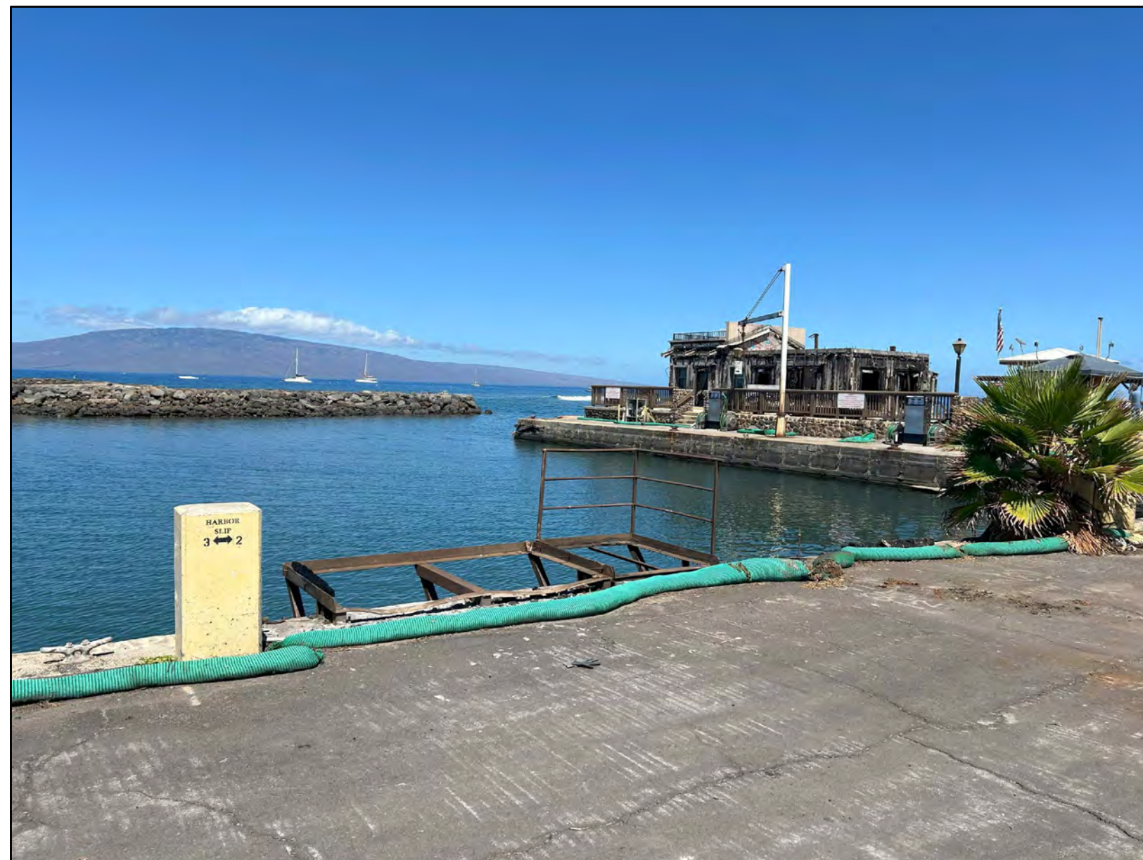
5 EXIST. METAL STRUCTURE TO BE REMOVED TAKEN 06/25/2024
