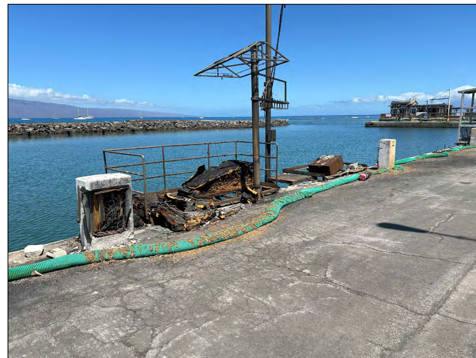
7 EXIST. METAL STRUCTURE AND DEBRIS TO BE REMOVED TAKEN 06/25/2024
