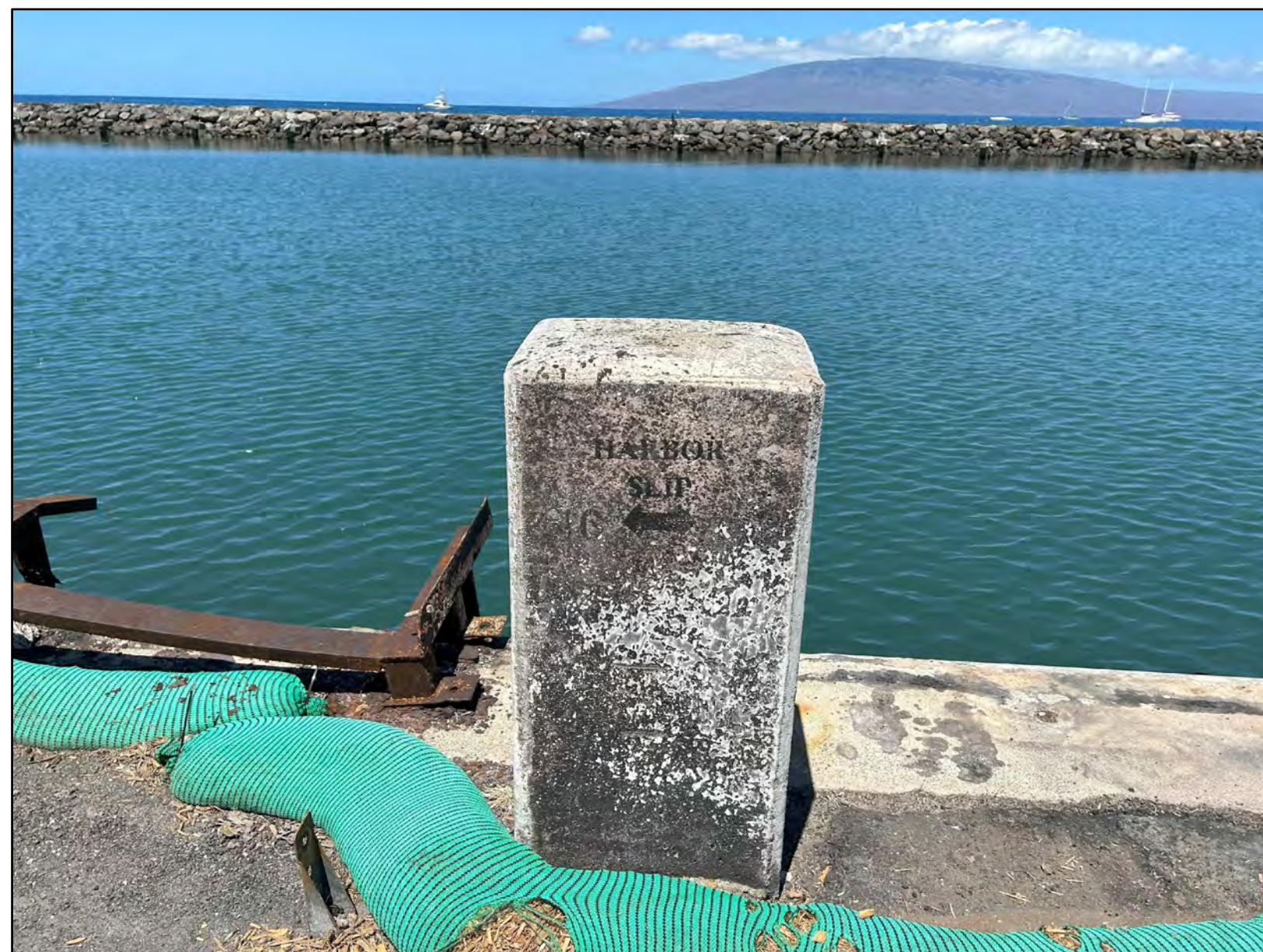
5 TYPICAL CONCRETE PEDESTAL TO REMAIN TAKEN 06/25/2024
