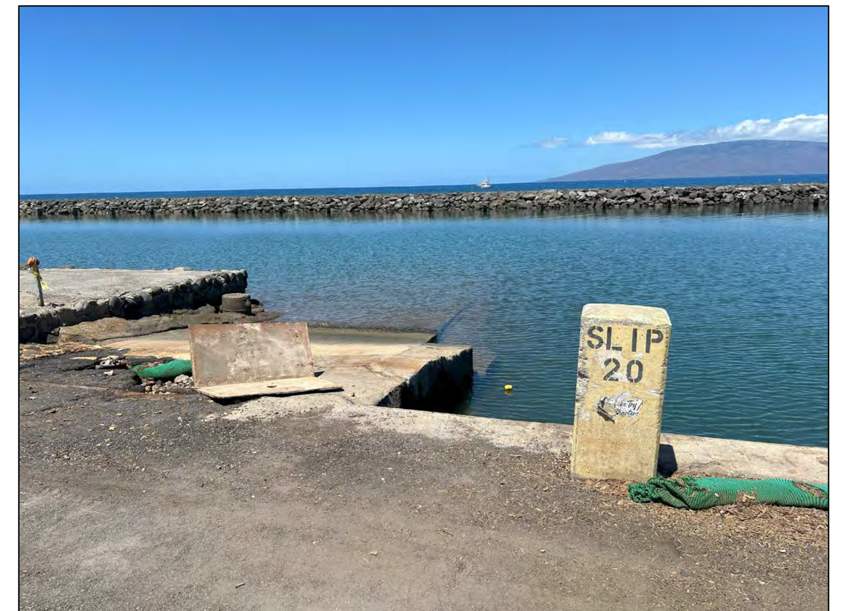
6 CONC. BOAT RAMP (SOUTHERN END OF FRONT ROW) TAKEN 06/25/2024
