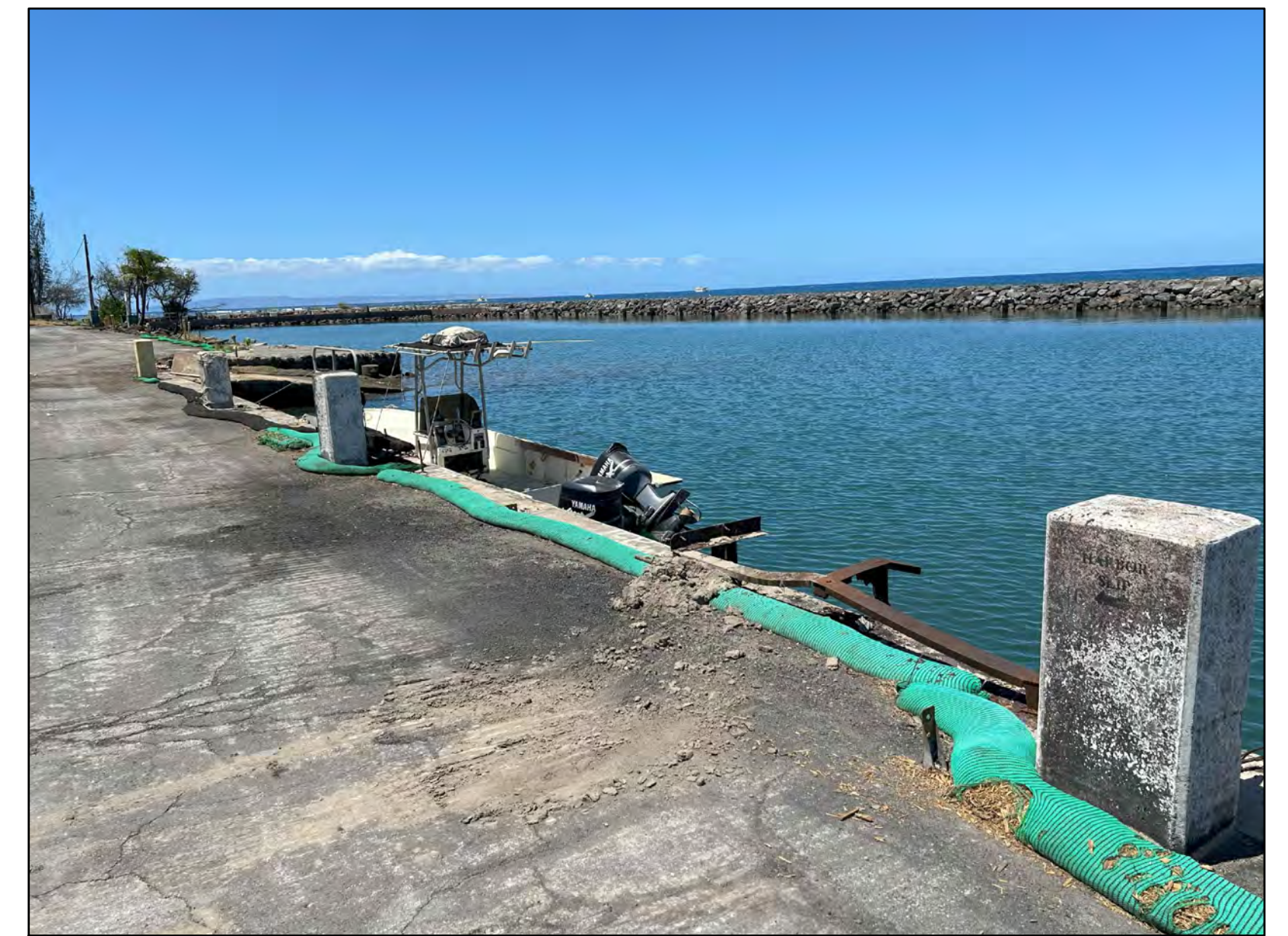
3 EXIST. CONDITIONS ON SOUTHERN SIDE OF LAHAINA SBH, FRONT ROW TAKEN 06/25/2024
