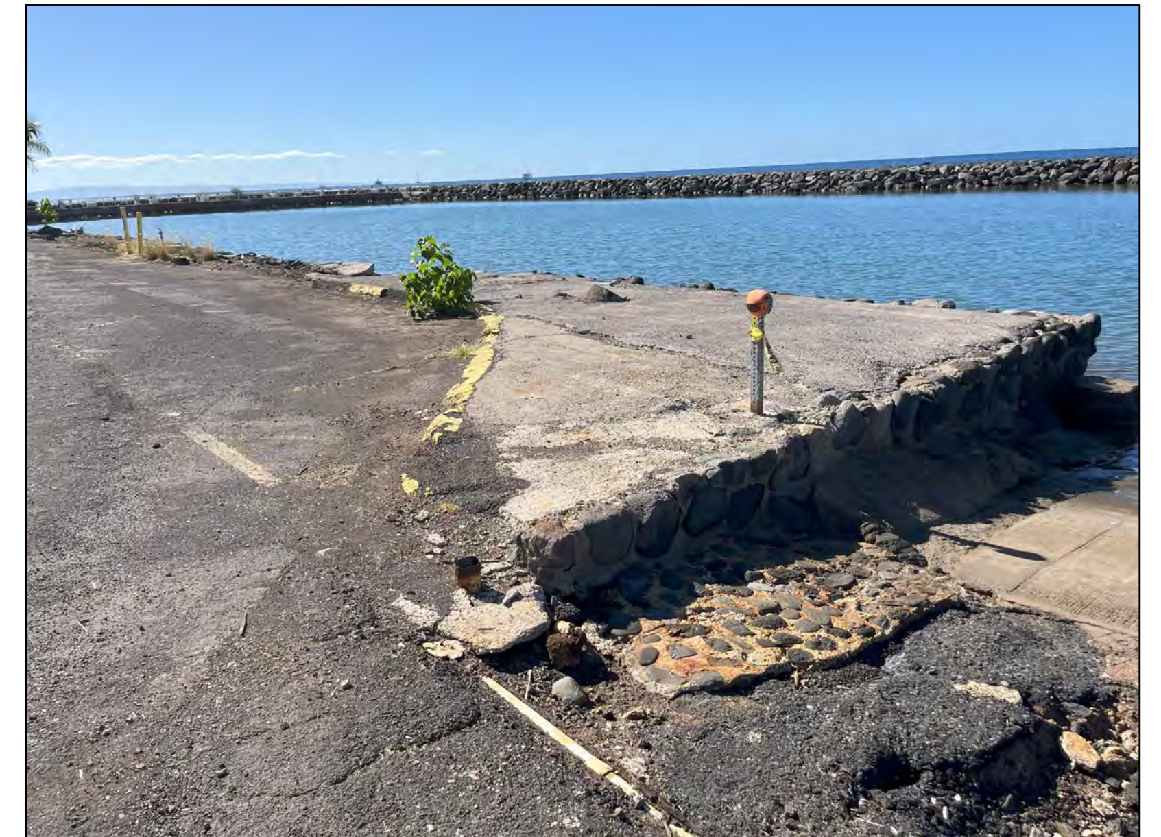
6 AREA ADJACENT TO EXIST. BOAT RAMP TAKEN 01/21/2025
