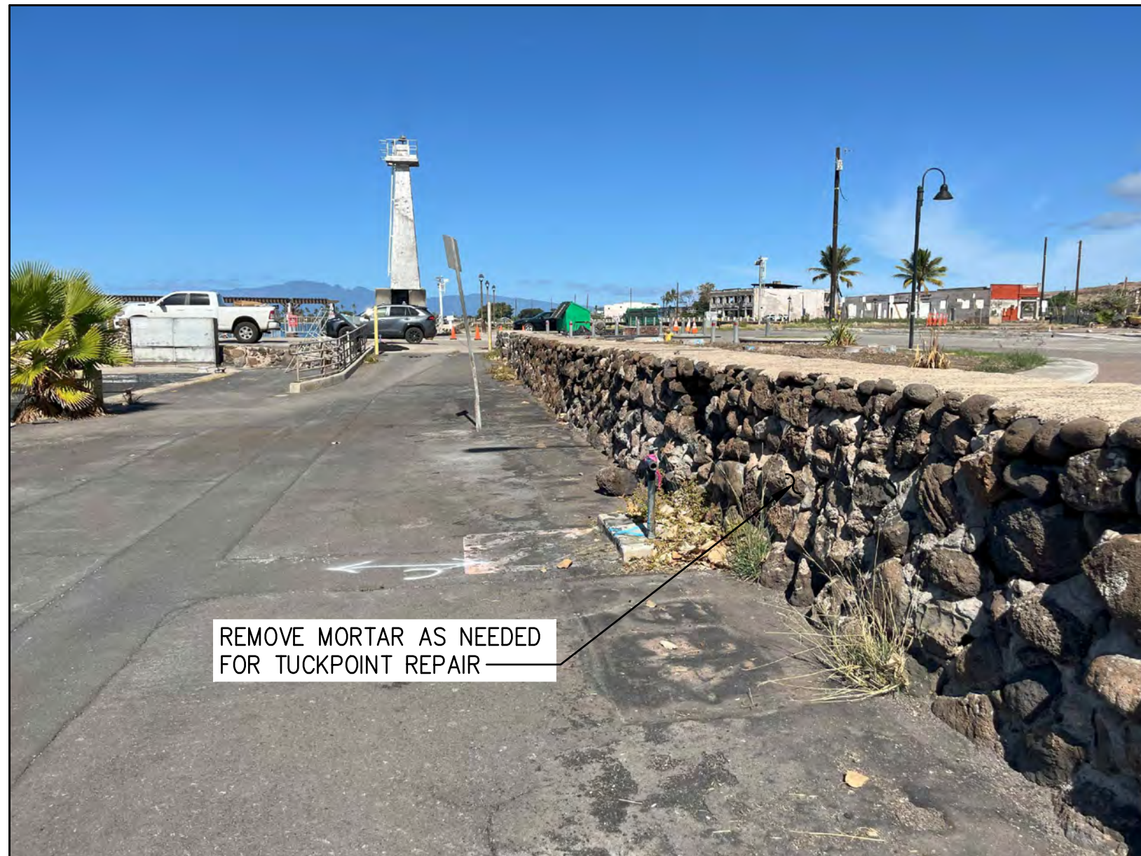
4 EXIST. CRM WALL (FACING SOUTHERN END OF FRONT ROW) TAKEN 01/21/2025
