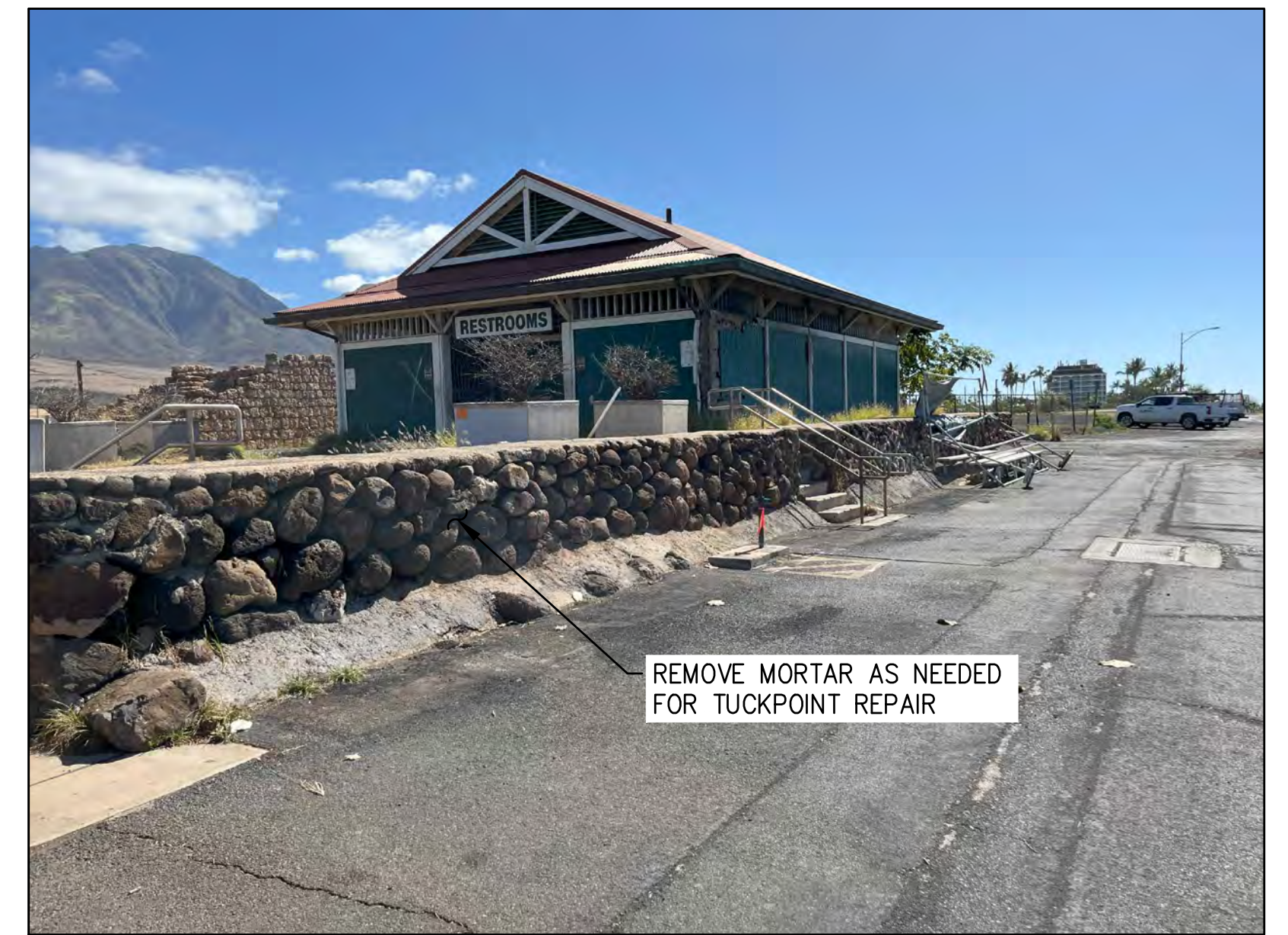
3 EXIST. CRM WALL (FACING SOUTHERN END OF FRONT ROW) TAKEN 01/21/2025
