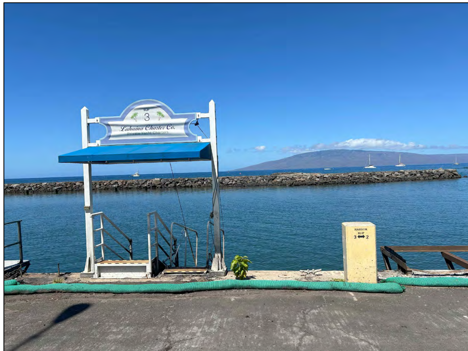
4 EXIST. METAL STAIRS & RAMP TO BE REMOVED TAKEN 06/25/2024
