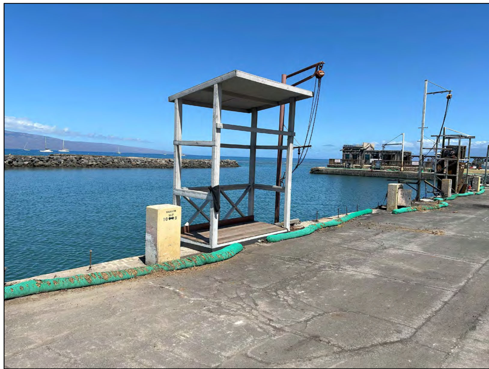
1 EXIST. WOODEN STRUCTURE TO BE REMOVED TAKEN 06/25/2024
